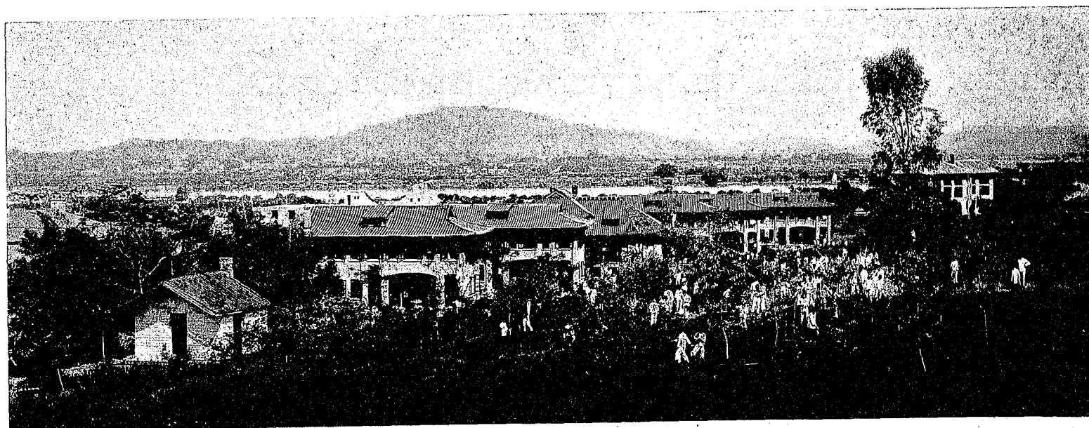
Primary School Cottages
