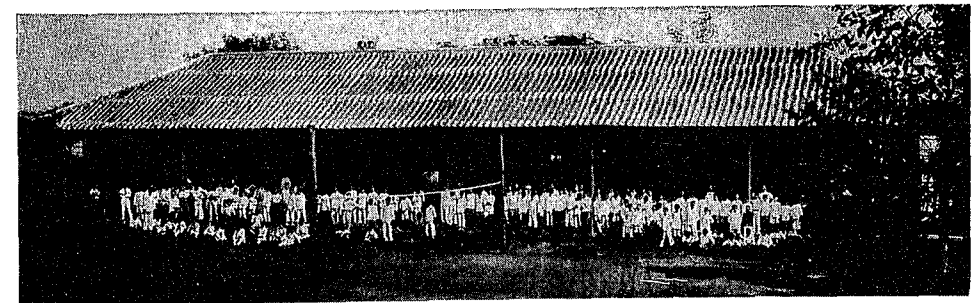
Temporary primary school building constructed of large gray brick from the city wall of Canton. When the wall was demolished the city authorities gave the brick to the College.
